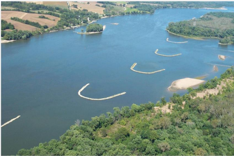
Upper Mississippi River Training Structures: Chevrons
